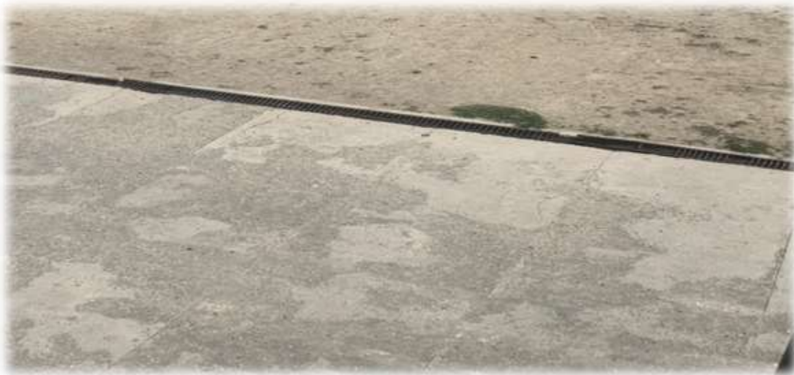
Caption: According to the provided image, the concrete surface of the runway section of the football stadium which has sustained damage. We aim to repair and rehabilitate this area.
